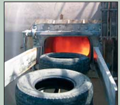
Mid Kiln Injection of Waste Tires
